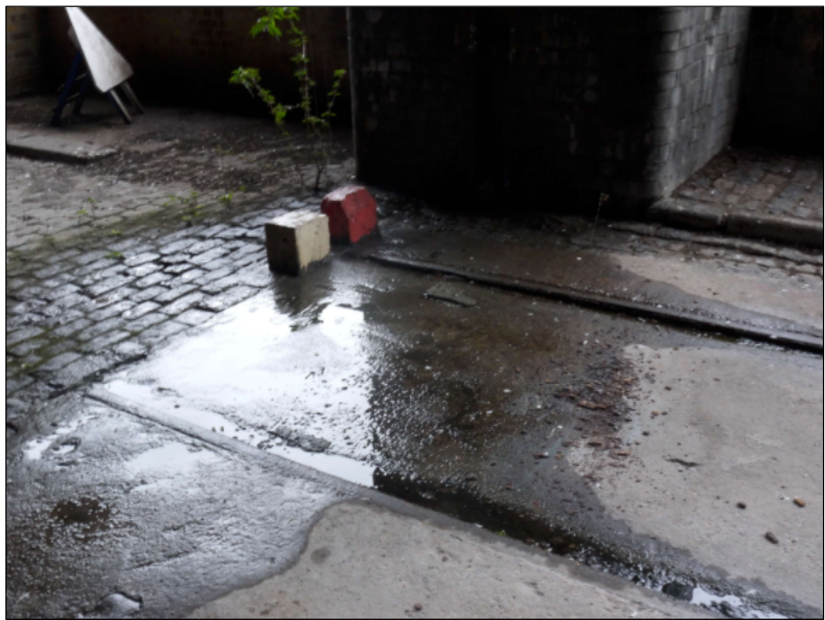
EXAMPLES OF VARIATION IN FLOOR LEVEL AND FINISH - It is proposed to construct new floor slabs in excavated units to bring shop units up to same level as the existing London Road Level. Existing hard landscaping materials in London Road (cobble, setts, railway lines etc) to be lifted and relaid. Refer to Spacehub drawings for proposals. Ramps in yellow to be removed
